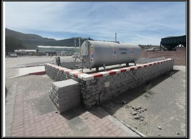
Bund wall repaired and sealed
